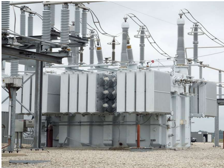
\Delta/Y_g —High Voltage Transformer
